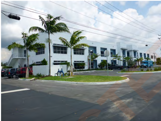
South curb cut & loading/parking area
