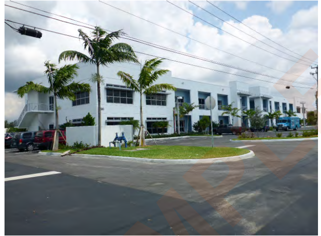
Dock-floor level rear connector (office right, studio B ahead, studio A to rear)
