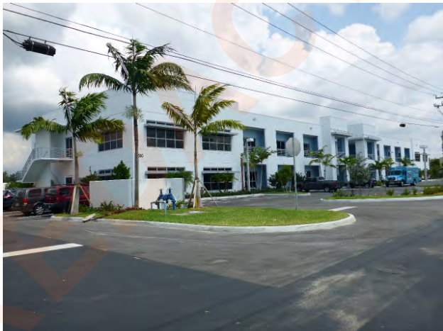
Typical dock level office
