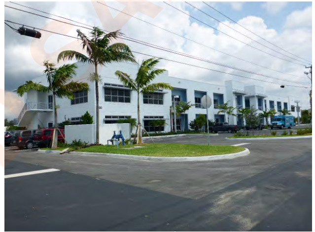
South on SW 18 th Avenue (subject right)
