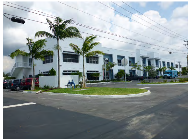
Front court (south to north)
