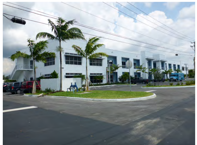
East on SW 184 th Street (subject right)
