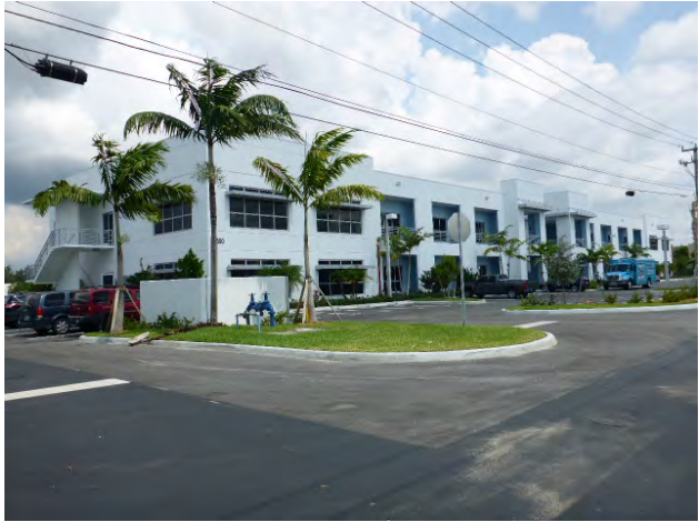
Stairway to second floor (one of two)
