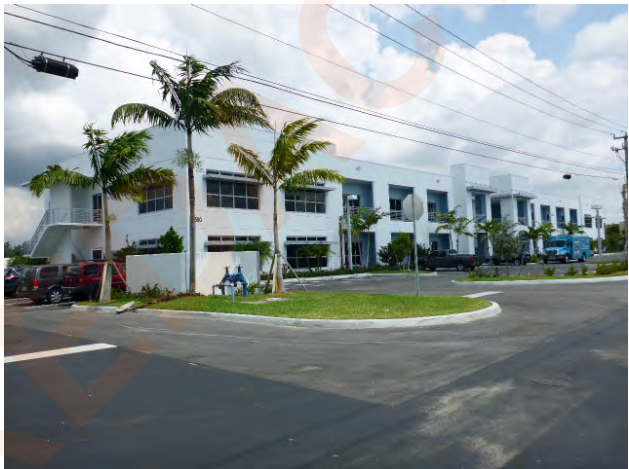
Second floor front office overlook
