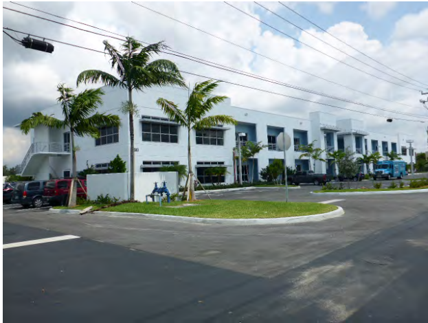
SEC of subject (south curb cut)
