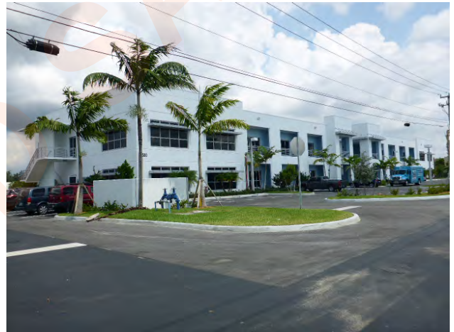
North curb cut & loading/parking area
